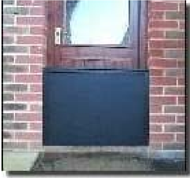
Figure 2. Flood barrier across external door ( http://www.antiflood.com/ )
